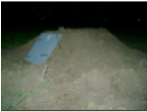
Frontal View of Completely Installed Shelter
