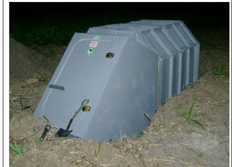
Shelter Assembled in 4-foot hole.
